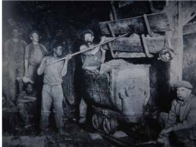
Mined ore, loaded from the ore pass into a cocopan.
