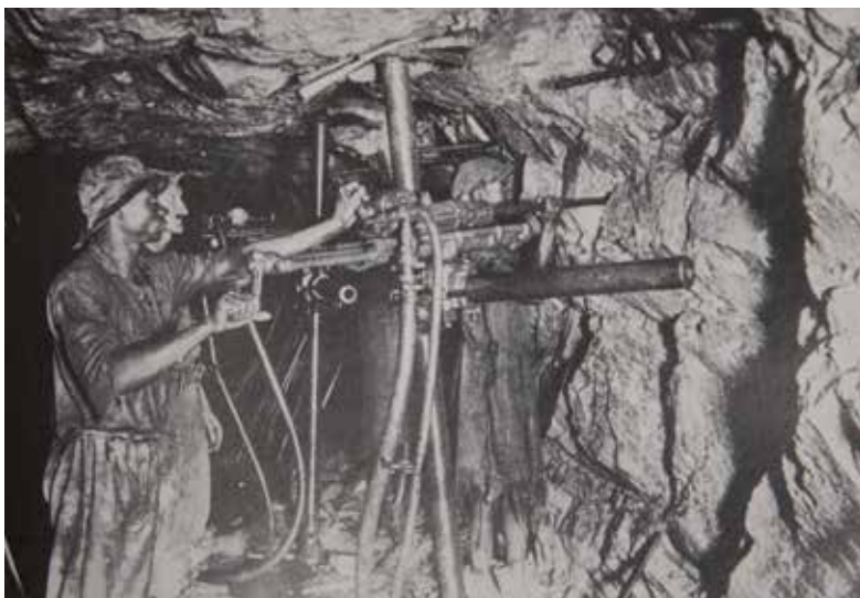
Drilling the rock face in preparation for blasting.
