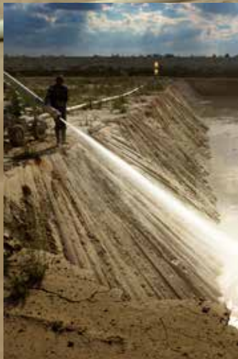
Reclamation of mine tailings by high-pressure water jet.
