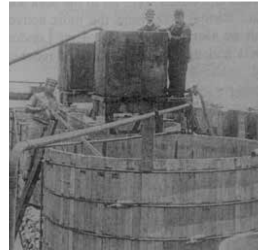
Early wooden cyanidation tanks used as part of the gold extraction process.
