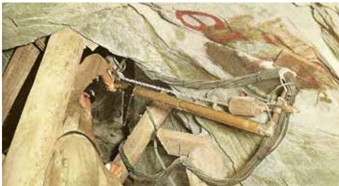
Hydraulic and pneumatic drills became more heavy duty to drill the rock face more efficiently.
