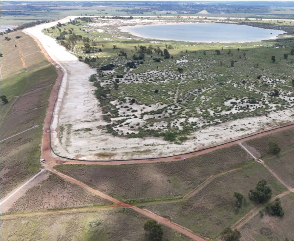
Aerial view of rehabilitation alongside active tailings retreatment at Ergo - Daggafontein TSF
